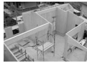
Fig. 8 – X-Lam Panels Structure
