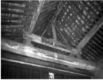
Fig. 3 – The Beam in Tiers Structural System
