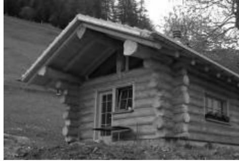
Fig. 2 – The blockbau system
